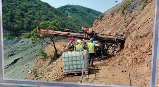
Self-drilling passive anchors, slope stability rehabilitation, Hydro-waste dump No.4, Sasa
