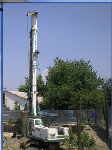
Residential building TRIM, Skopje
