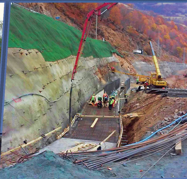
Prestressed active anchors, landslide Kalimanci, State road Kocani-Delcevo
